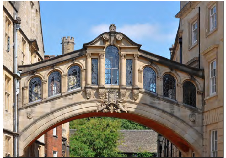
Hertford Bridge (aka, "The Bridge of Sighs")
